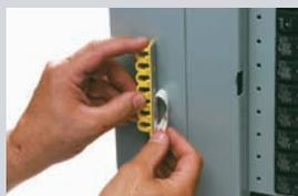
1. Expose the super-bond adhesive on back of rail. Permanently affix to any location on the panel.
