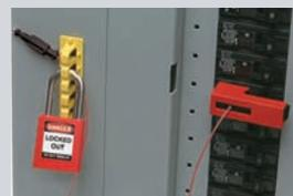
3. Pass plastic key through lock rail and attach lock, preventing key from sliding down cable to device.
