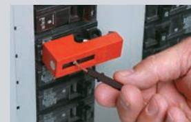
4. After procedure is finished, unlock device by inserting and turning the black plastic key.
