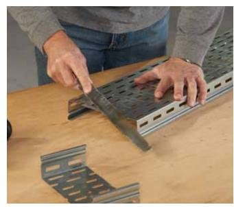
CUTTING STRAIGHT SECTIONS FOR ELEVATION CHANGES
