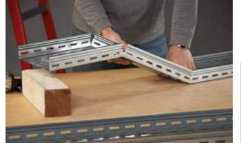
To splice straight sections of V-Trough use the FTEF. The FTEF has attachment hardware included and should be used when splicing V-Trough straight sections or fittings.
