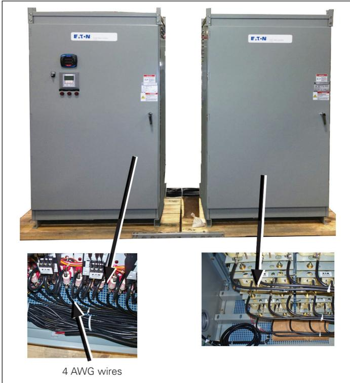
Figure 6. Current transformer wiring for IQ Meter
