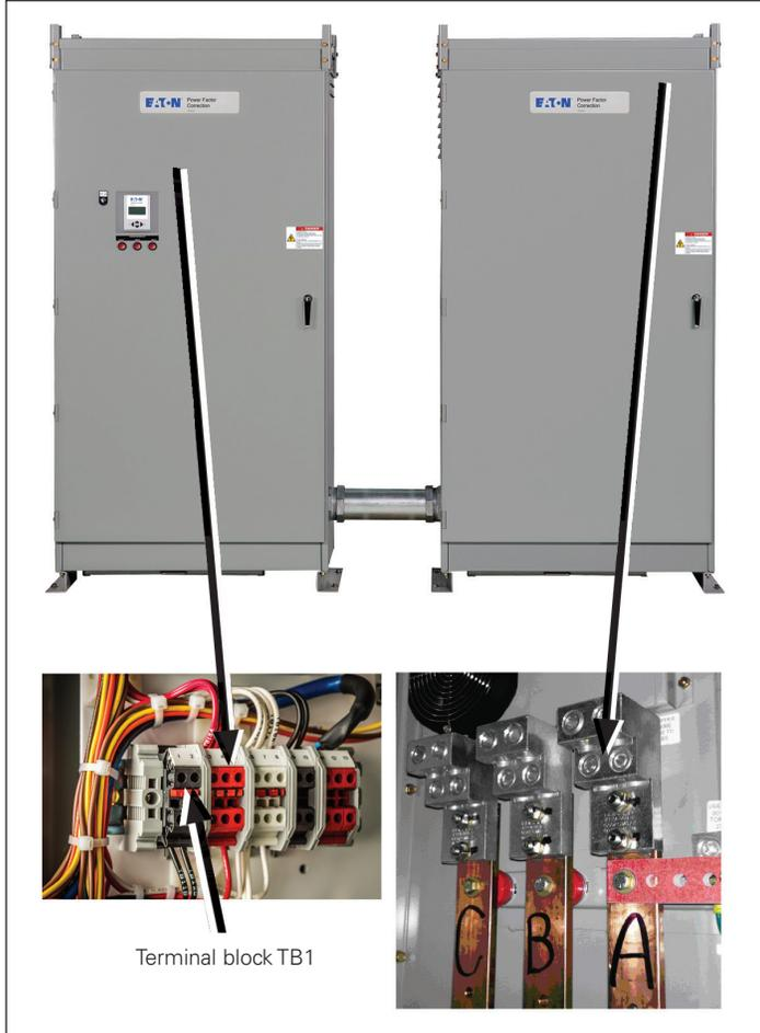
**Figure 3. Current transformer and power wiring termination points**
