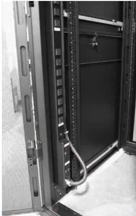
Power Commander Plus High Current Power Distribution Unit shown mounted in an IT cabinet.
