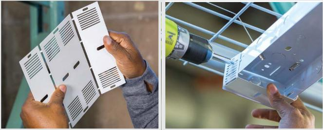
**STEP 4:** Connect power from building to quick disconnect on retrofit kit. Bring retrofit kit up to fixture frame.
