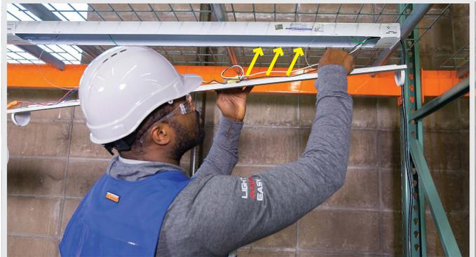
**STEP 5:** Fasten the pans to the strip fixture with a quarter turn (provided) on each end.
