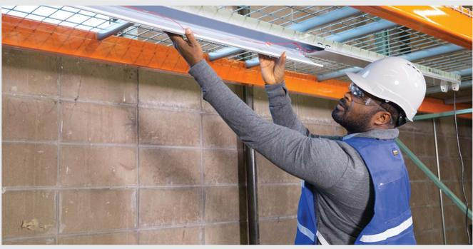
**STEP 2:** Cut the wire leads coming from the sockets and remove the sockets and socket bars on both ends of the fixture.
