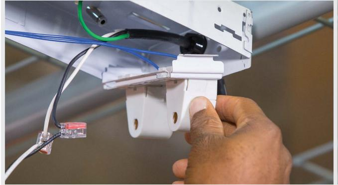
**STEP 3:** Break apart the 1-piece mounting bracket kit into 3 individual pieces. Install a small bracket at each end of the fixture and the large bracket at the center of fixture (for 8' fixtures only). Bend the brackets over the fixture to fit the exact width and fasten them to the fixture with the provided tek screws.
