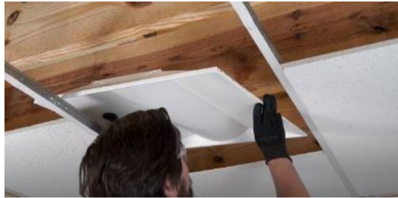
Position the lay-in in the ceiling grid
