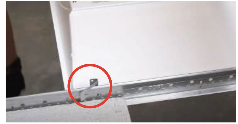
Attached all 4 t-bar clips
