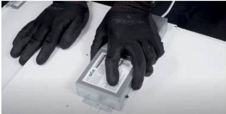
Select switchable settings, insert the driverbox on the back of the fixture
